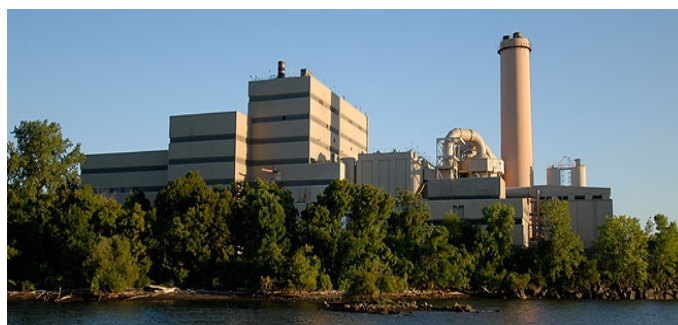
Wheelabrator Westchester L.P. Waste-to-Energy Facility (Source: http://wheelabrator technologies.com/plants/waste-to-energy/wheelabrator-westchester-lp/ )
