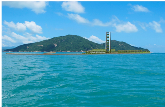
A Photomontage showing the Government's Proposed IWMF on the Artificial Island off SKC. It is prepared based on the figures in the Legislative Council Brief titled "Development of the Integrated Waste Management Facilities" by EPD, February 2011.
